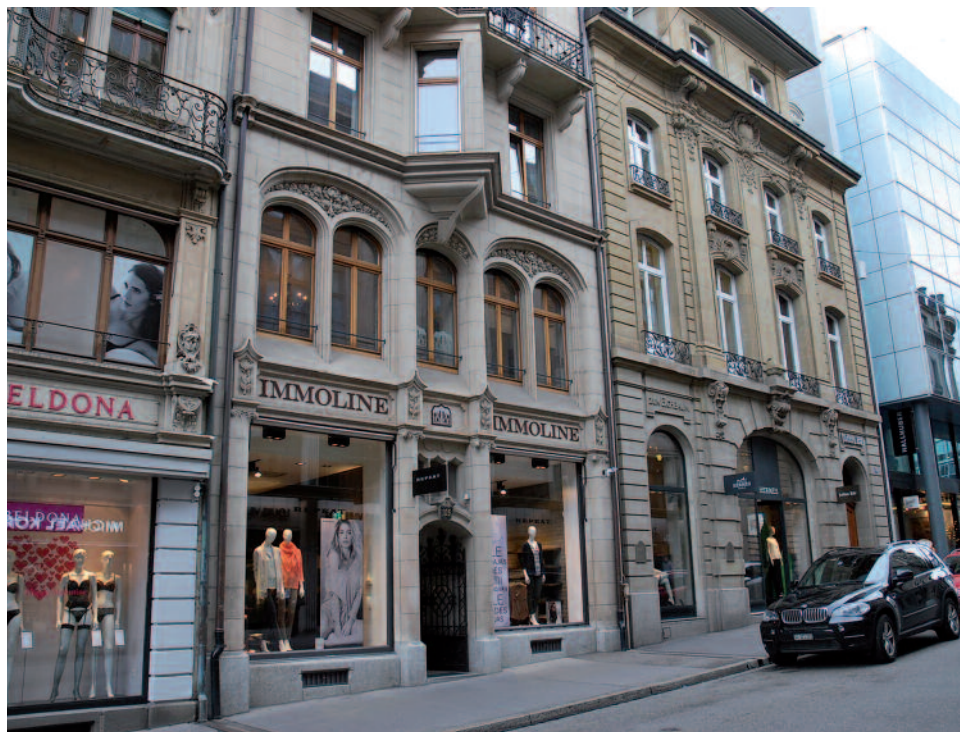
Immoline-Office, Freie Strasse 105
